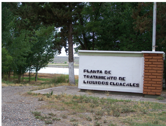
Photo 4. Urban Waste Water Treatment Plant of Obras Sanitarias Mendoza in Tunuyán; the treatment pools are behind the trees.
